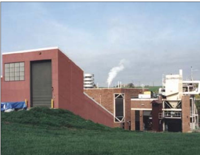
Demonstration Boiler Facility
